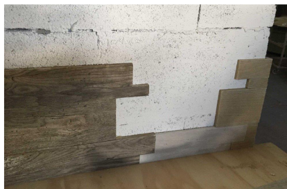
7. Working from the bottom to the top, right to left install the next row of panels until the gap between the corner piece and the full panels is less than a full panel.
