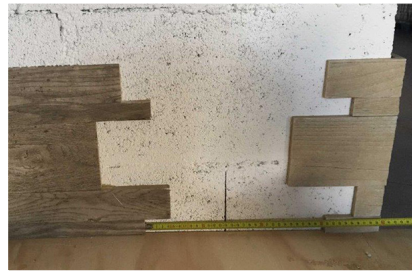
2. Work from left to right by installing Antique Wood panels until the gap between the corner pieces and full panels is less than a full panel.
