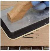
Use a flat wood block or rubber grout float to beat the face of the tiles and firmly embed the tiles into the mortar.
