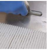
Using the appropriate sized small square notch trowel, add more adhesive and notch the mortar in a horizontal, straight pattern.
