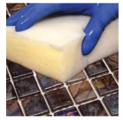
Within one hour of initial set, clean any residual glue and paper from the surface using a light, damp sponge and buff with a dry cloth.
