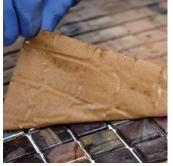
When the paper is properly saturated, peel the paper from the face of the tile being careful not to pull tile away from the mortar. Two or more applications of water may be needed to safely remove the paper facing from the tile.
