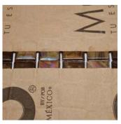
Place the glass mosaic sheets onto the fresh mortar and bring all surfaces to a true plane at the proper position.
