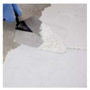
Key the mortar into the substrate using the flat side of a trowel to initiate a bond coat.
