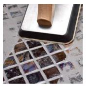
Apply grout with a rubber grout float, forcing grout into joints until full.
