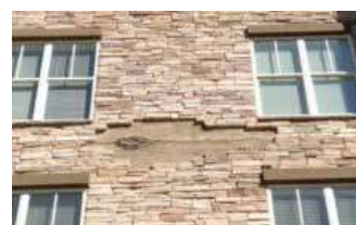
Adhesion Failures
