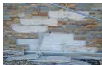
Delamination of Stone
