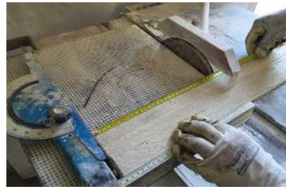
5. Cut down the individual pieces from step 4 to fit the gaps you measured in step 3.
