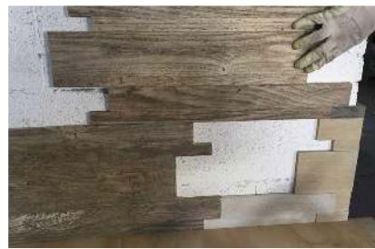
8. By alternating the installation on your wall, starting one row on the left and the next row on the right, the installer ensures that the rows are always slightly offset, thus providing seamless final installation.
