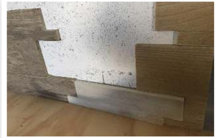
6. Install the individually cut pieces into the gap.
