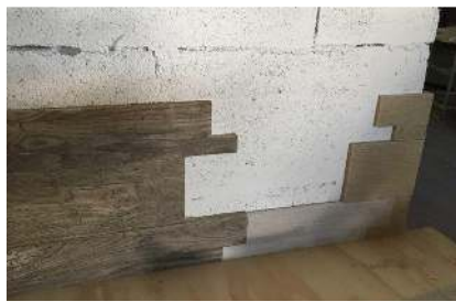
7. Working from the bottom to the top, right to left install the next row of panels until the gap between the corner pieces and the full panels is less than a full panel.
