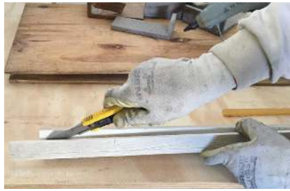
4. Use a sharp industrial knife to cut the mesh at the back of each panel so you end up with individual loose pieces.
