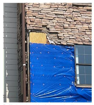
Tradition last and scratch installations are vulnerable to moisture, leading to failures as seen above.
