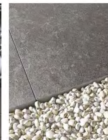
Dry-lay on gravel
